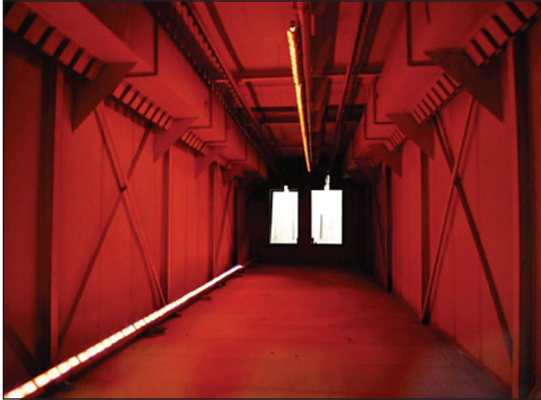
A look inside our oven after the new burners were installed
